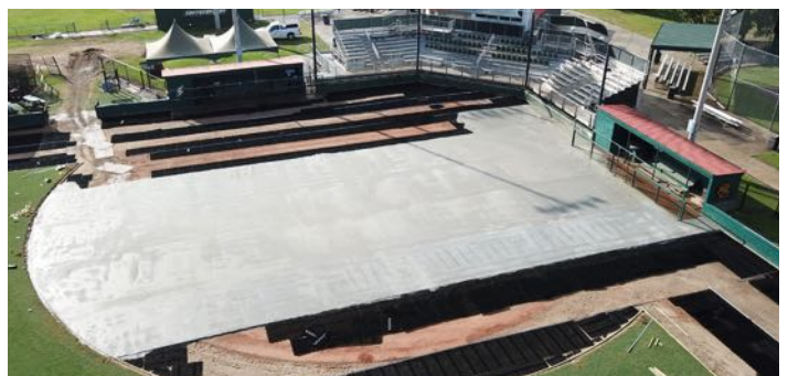
READY TO INSTALL TURF AFTER DRYING
