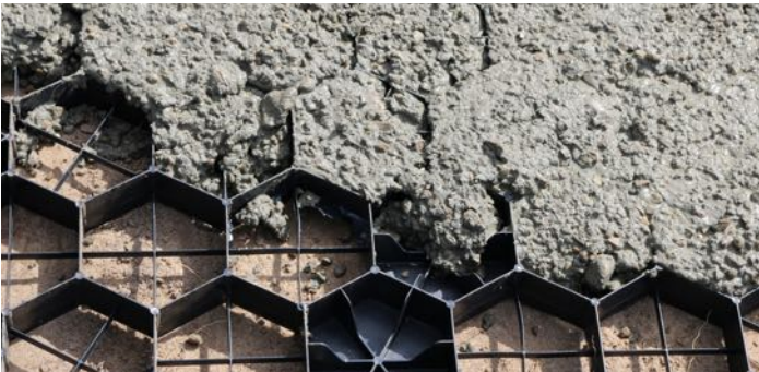
CONCRETE POURING OVER GRID
