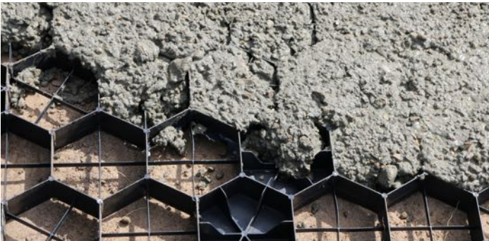
CONCRETE POURING OVER GRID
